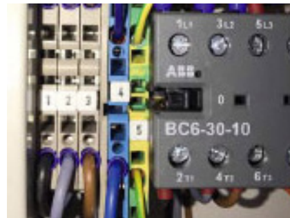
3 Phasen / 3 phases 1 - 2 - 3 Neutral / neutral - 4 Erdung / earth - 5
